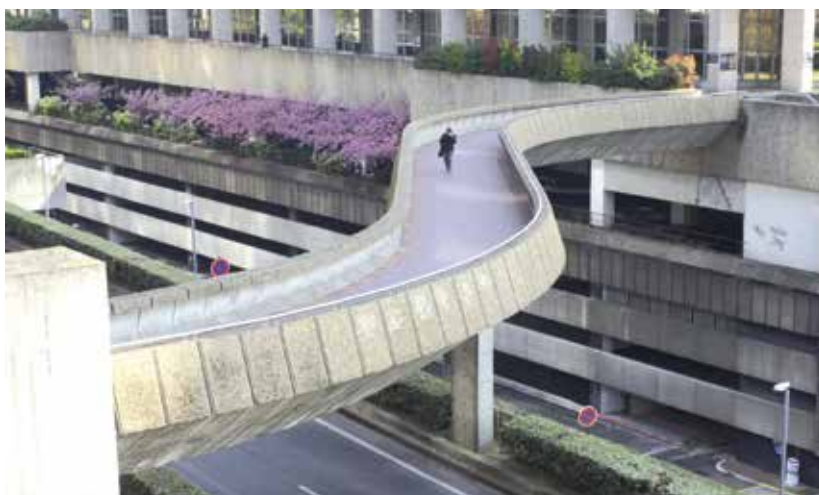
Passerelle Jean Moulin, photographie, 2013, service Communication.
