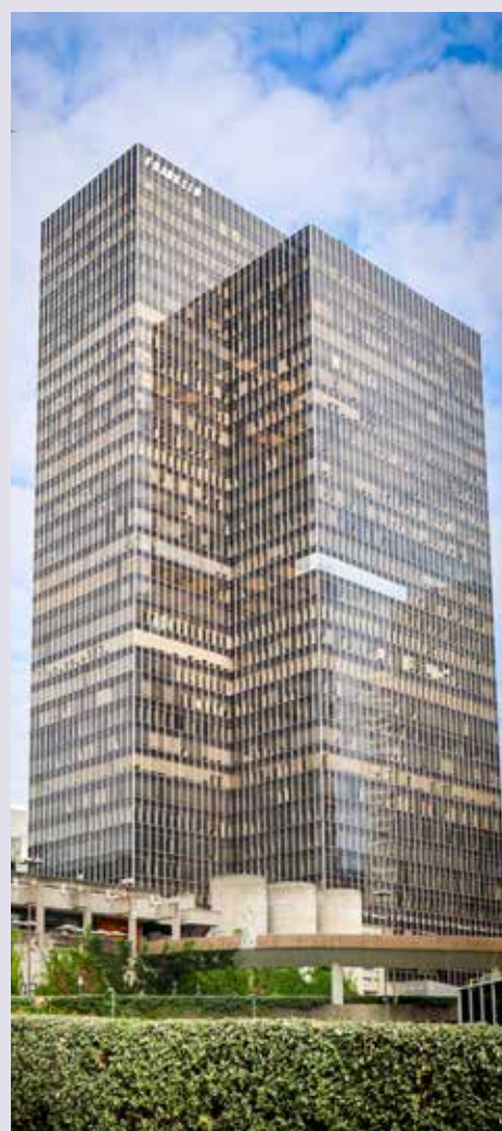
Tour Franklin, photographie, 2026, service Communication.
